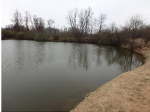
Pond PMO-JJP-003, Facing North (3/16/17)
