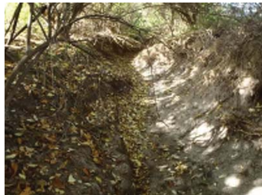
Stream SIL-CDK-003, Downstream, Facing West (11/1/16)
