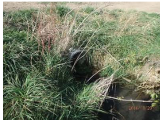
Stream SIL-TMA-078 Downstream, Facing West (11/20/16)
