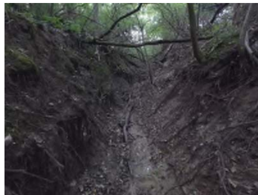
Stream SIL-TMA-016, Downstream, Facing South (9/12/16)
