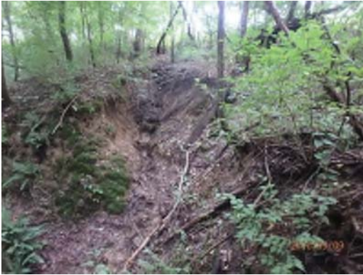
Stream SIL-TMA-006, Upstream, Facing Southwest (9/9/16)
