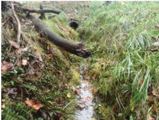
Stream SIL-CDK-013, Upstream, Facing West-Northwest (11/3/16)
