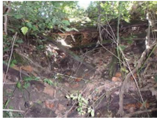
Stream SIL-TMA-012, Downstream, Facing Northwest (9/12/16)
