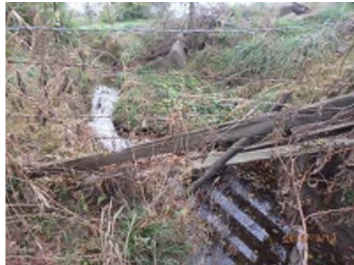
Stream SIL-TMA-042, Downstream, Facing West (10/19/16)
