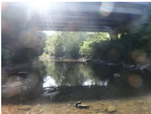
Stream SMO-DFW-008, Upstream, Facing West (9/20/16)
