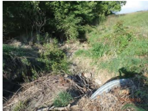
Stream SIL-TMA-023, Downstream, Facing East (9/15/16)
