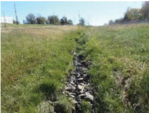
Stream SMO-CDK-004, Upstream, Facing South (11/10/16)
